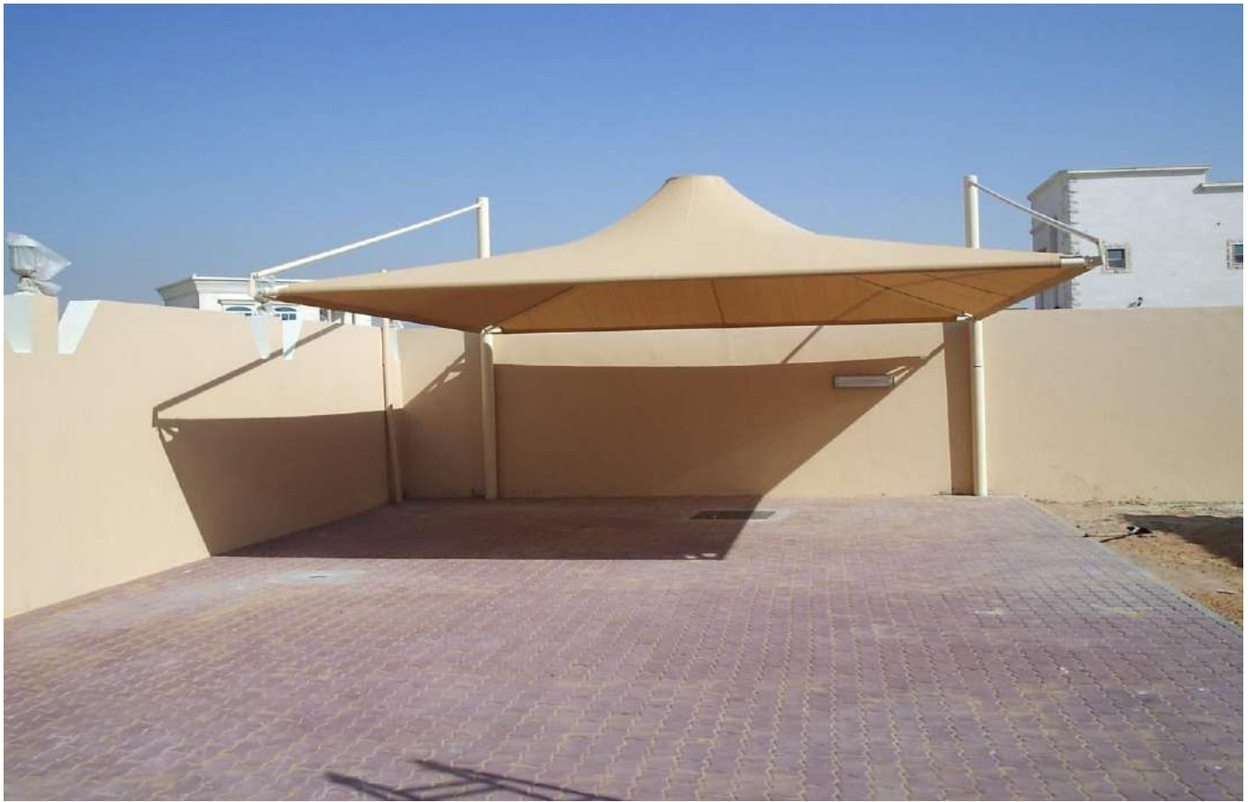
Car parking dome shape for two cars, DUBAI
