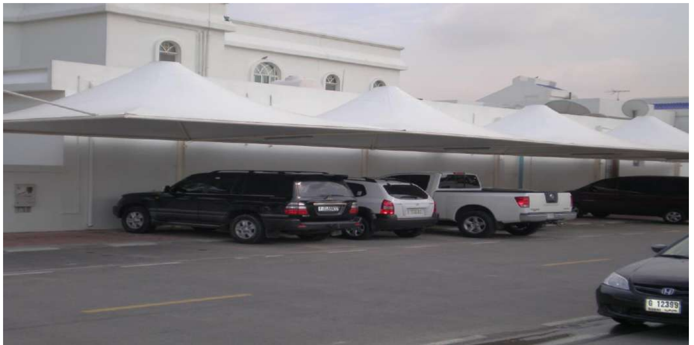
Car parking lot-Dome type, Mamzar Dubai, UAE
