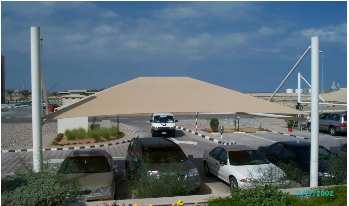
Car parking for three cars, Mesaeed, Qatar
